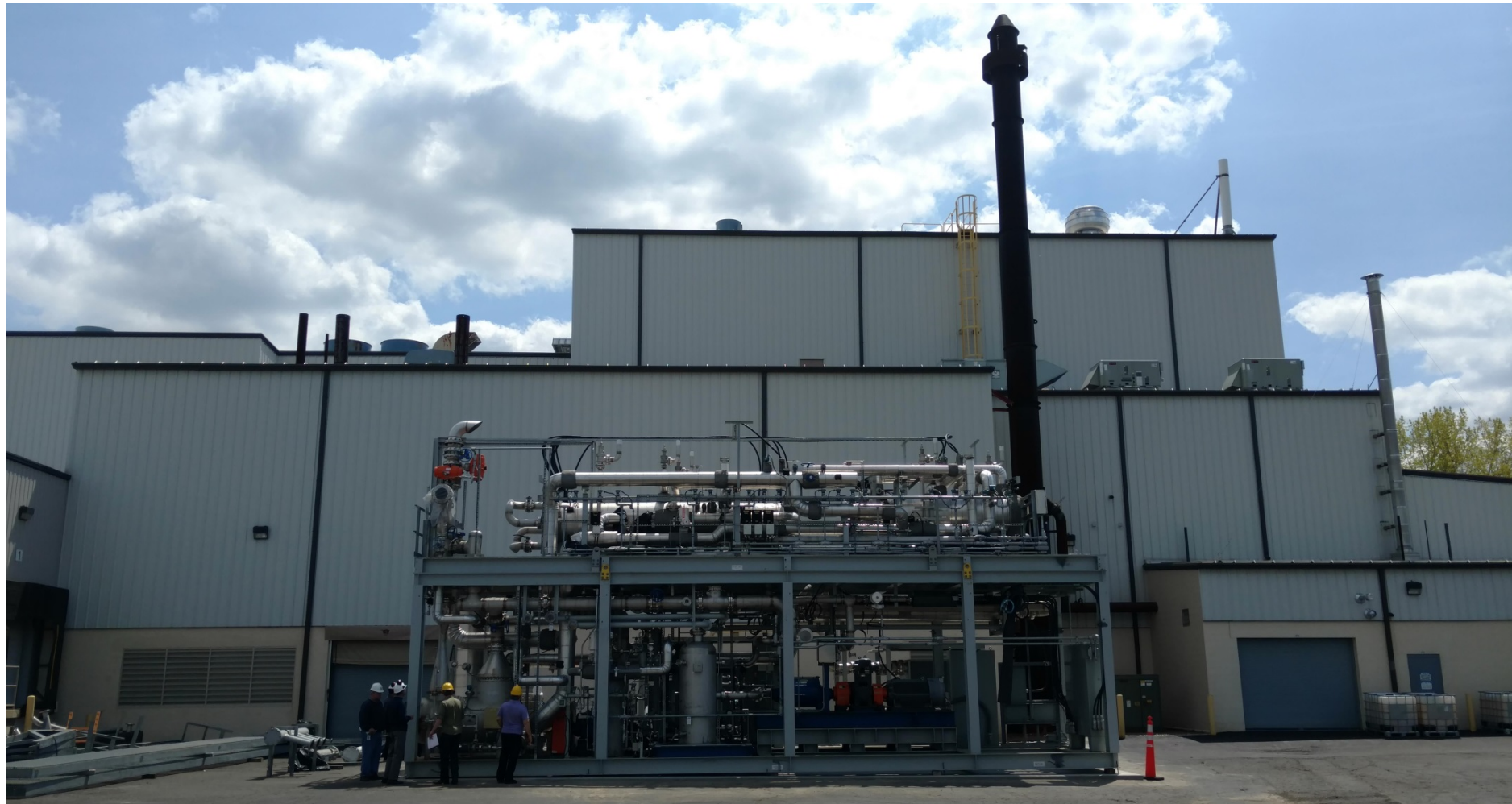
Skid with B&W 0.6 MW e SBS-II boiler facility in background
